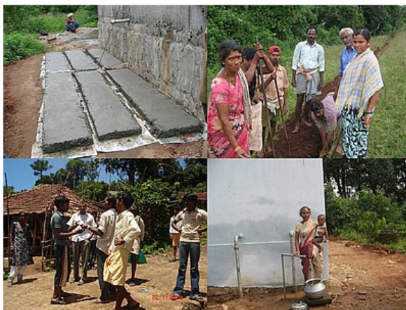
Completion of Construction Work at Rintada Photo credit: Apalanaidu, VJNNS
